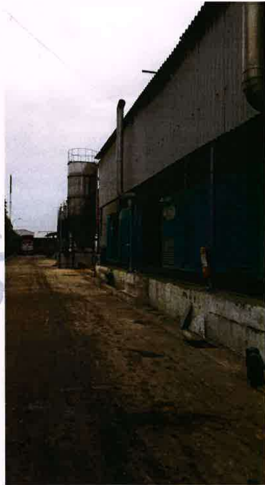
Silent Diesel generators
