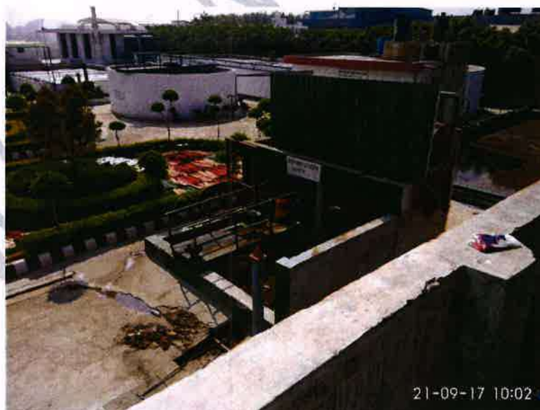
Modern effluent treatment plant
