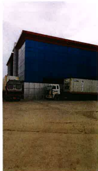
Slaughtering facility and refrigerated trucks
