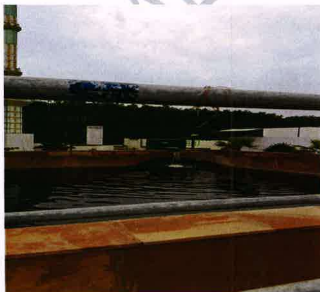
Clear water storage tank at the end of ETP.
