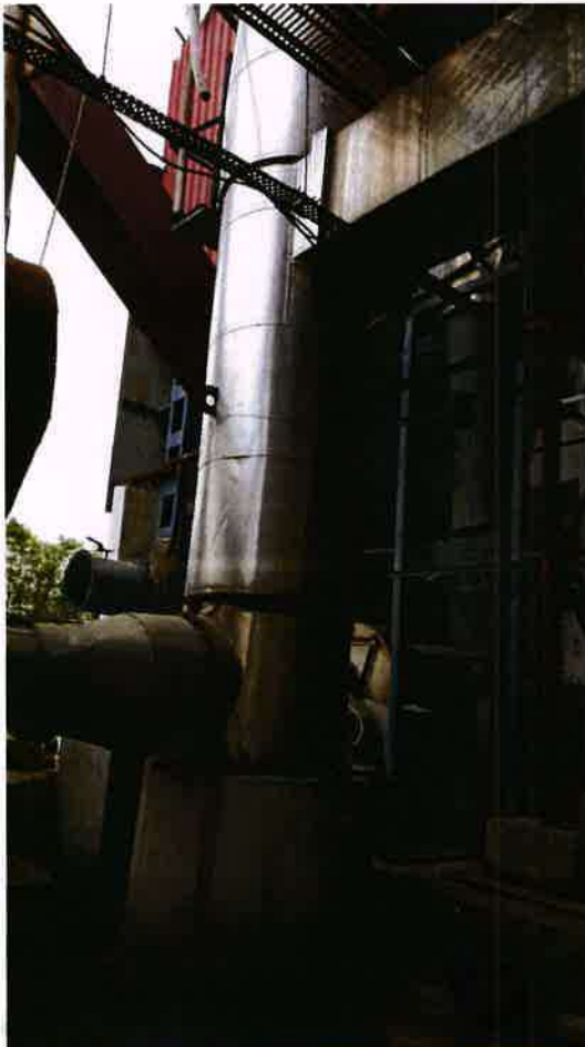
APCS and stack installed in the Boiler Fitted with online stack monitor
